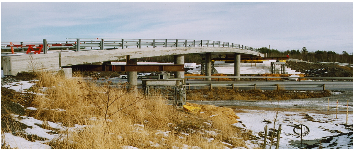
Figure 20. Temporary support of abutments at Hjelmungen
