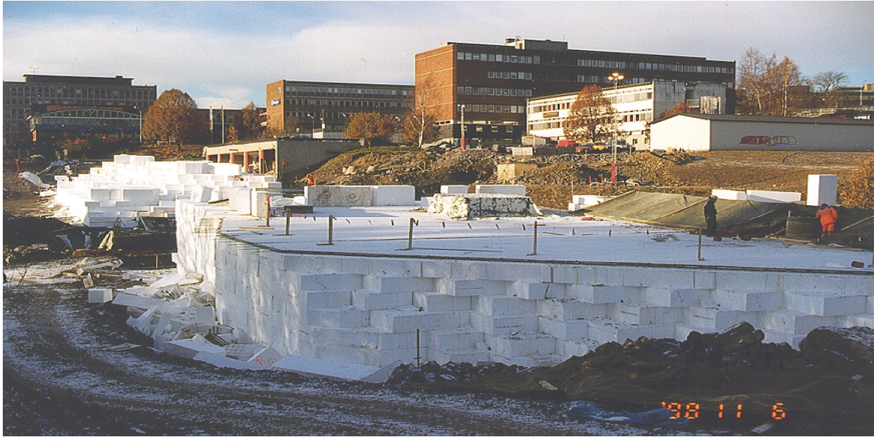
Figure 1. An EPS embankment for a city tramline in Oslo with vertical walls as an alternative to a bridge.
